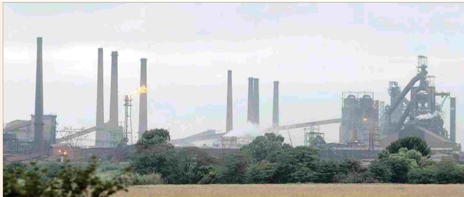
ArcelorMittal SA says dust emissions are at their lowest at its Vereeniging works, following the installation of a dust extraction system in 2010.
